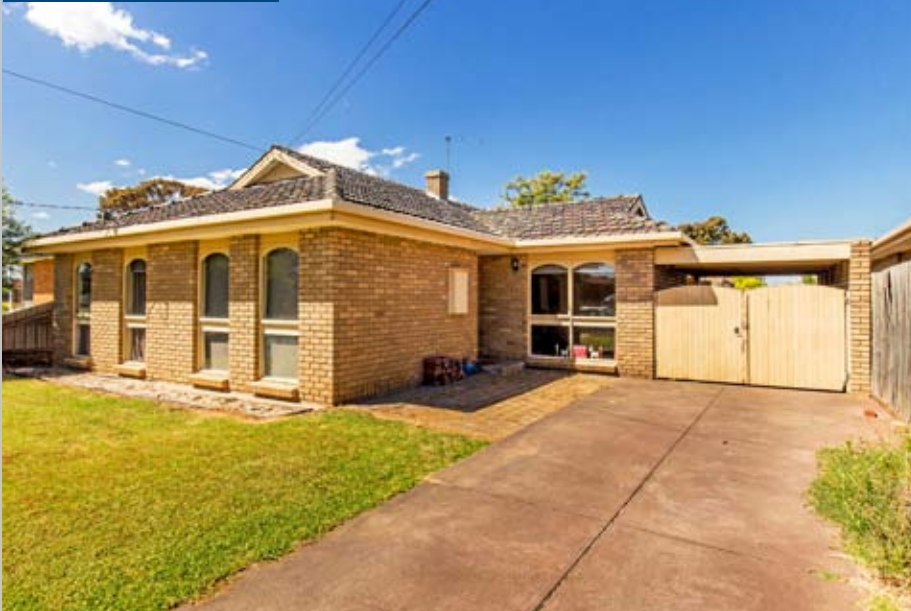
HOPPERS CROSSING 3 STRANG STREET
